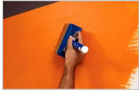
Step 4 - First coat by "pull and blend"
