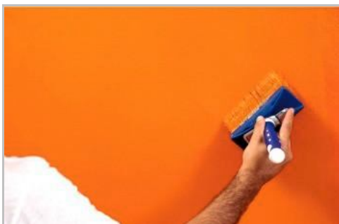
Step 5 - Second coat by "pull and blend"
