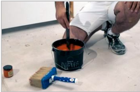
Step 3 - Mix the product until it's homogeneous
