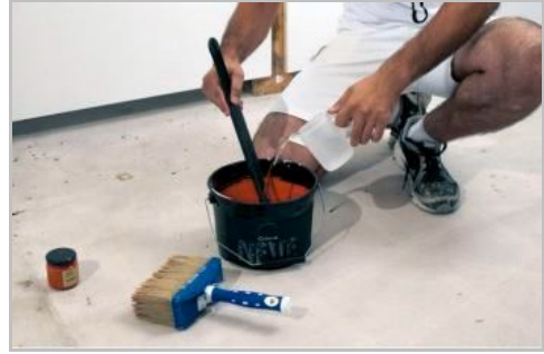
Step 2 - Prepare the shade with Neve and add 30% water solution.
