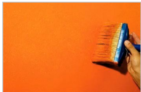
Step 6 - Third coat by "pull and blend"
