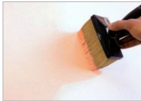
Step 4 - First coat by "pull and blend"
