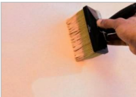
Step 5 - Second coat by "pull and blend"
