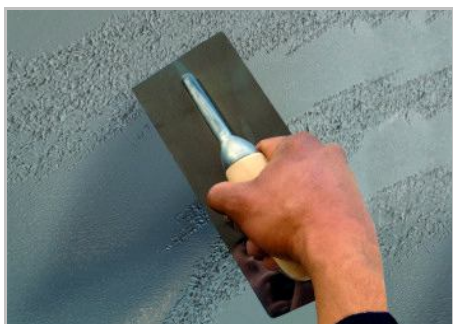
Step 5 - When the product begins to dry proceed with the compacting and polishing phases.
