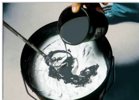
Step 2 - If needed, prepare the shade with our paints indicated in the sample collection and mix with the beater; allow to rest for 24 hours.
