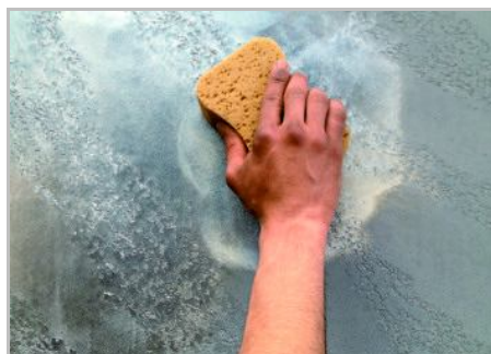
Step 6 - Obtain the desired finishing with Gioia, Oro, White Paint or Cera del Vecchio. If needed, increase the surface protection with Vetro-Frammenti.
