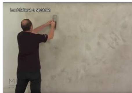
Step 6 - To get a stronger lucidity you can still pass our spatula for a dry polishing. If desired, give a protection with Savon d'Eau, Cera del Vecchio, Vetro Lucido or Opaco, according to the required breathability or resistance.
