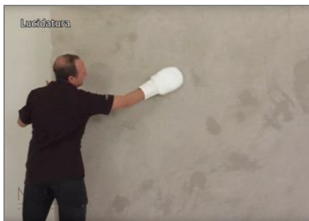
Step 5 - When the product lightens demonstrating that it is almost dry, polish the surface with a glove PE6.
