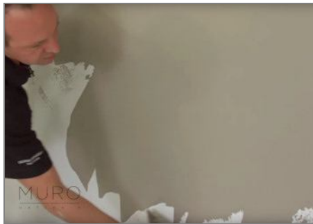
Step 3 - Applied in just one coat, freely distribute the product with the trowel.
